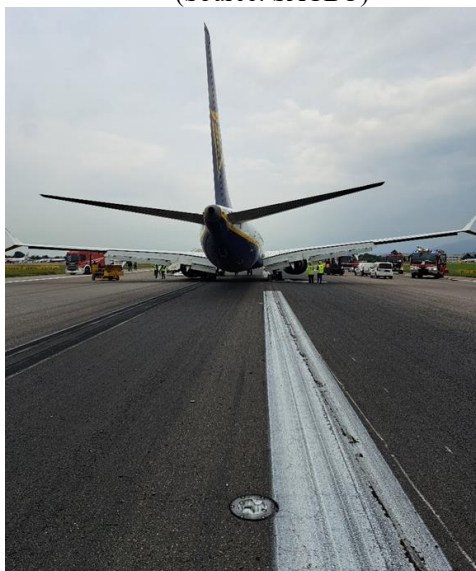
Photo 6 - area of the runway, near the aircraft, affected by damage and debris (Source: SACBO)
